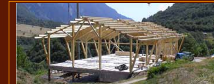
AGRICULTURAL BUILDING Switzerland 2003
